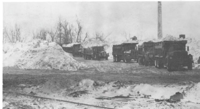
SNOW REMOVAL entailed trucks brought in to carry away huge piles of snow pushed or blown aside by plows or collected by front end loaders.
