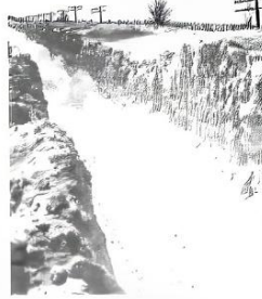
Despite the efforts of a rotary plow, eating through 21-foot drifts, this section of the Danville Branch, just north of Sheff, Ind., remained impassable.
